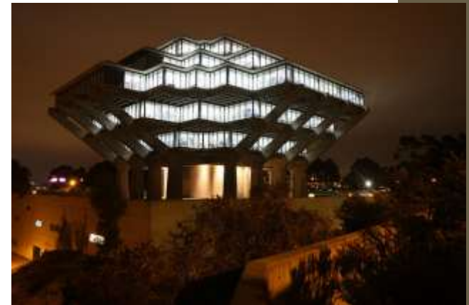
The Geisel Library at night, lit by locally-sourced microgrid energy | Photo: Nathan Rupert /Flickr/ Creative Commons License
