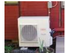
Ductless Heat Pump
